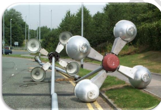
Figure 9.4 Maintenance of high mast lighting
