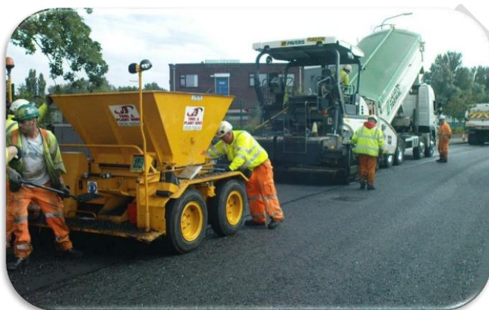
Figure 9.1 Carriageway resurfacing
